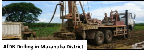
AfDB Drilling in Mazabuka District
